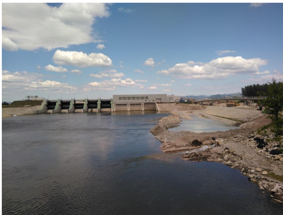
The Brežice hydropower plant on the river Sava in Slovenia. Photo taken by the author
