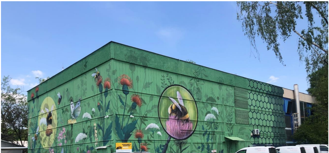
Geothermal heating plant in Szeged, Hungary
