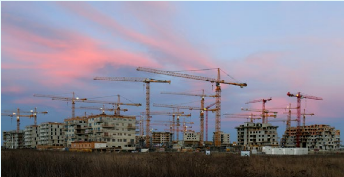
Figure 16 - Smart district of Aspern under construction (Source: Aspern Smart City Research)
