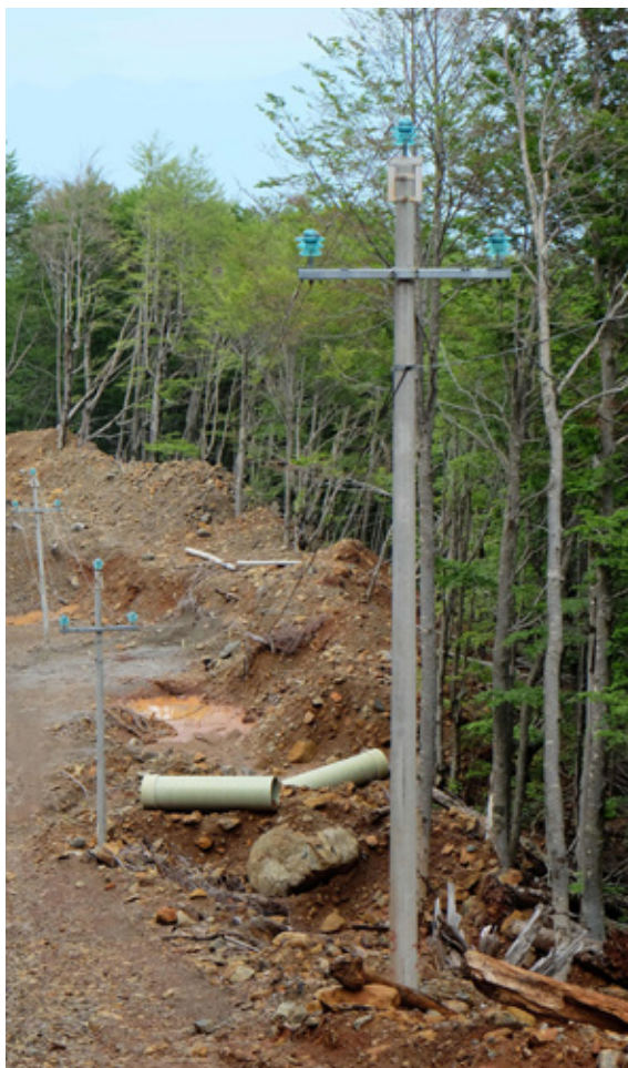
Figure 16: A section cleared for the access road and electricity poles
