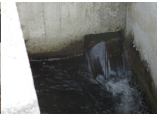
Figure 23: The upstream exit from the fish pass on Brajcinska intake
