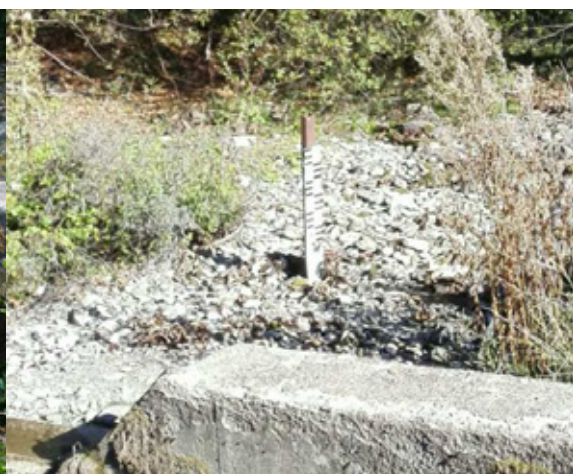
Figure 27: The weir above the powerhouse November 2017
