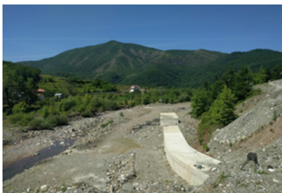
Figure 10: Tunnel taking tailwater to Rapuni 3 & 4
