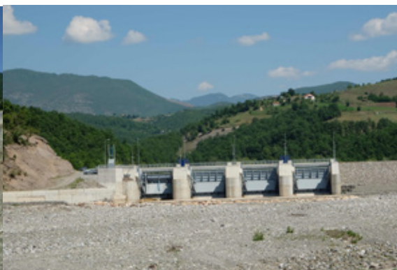
Figure 11: Rapuni 3 & 4 dam leaves no residual flow
