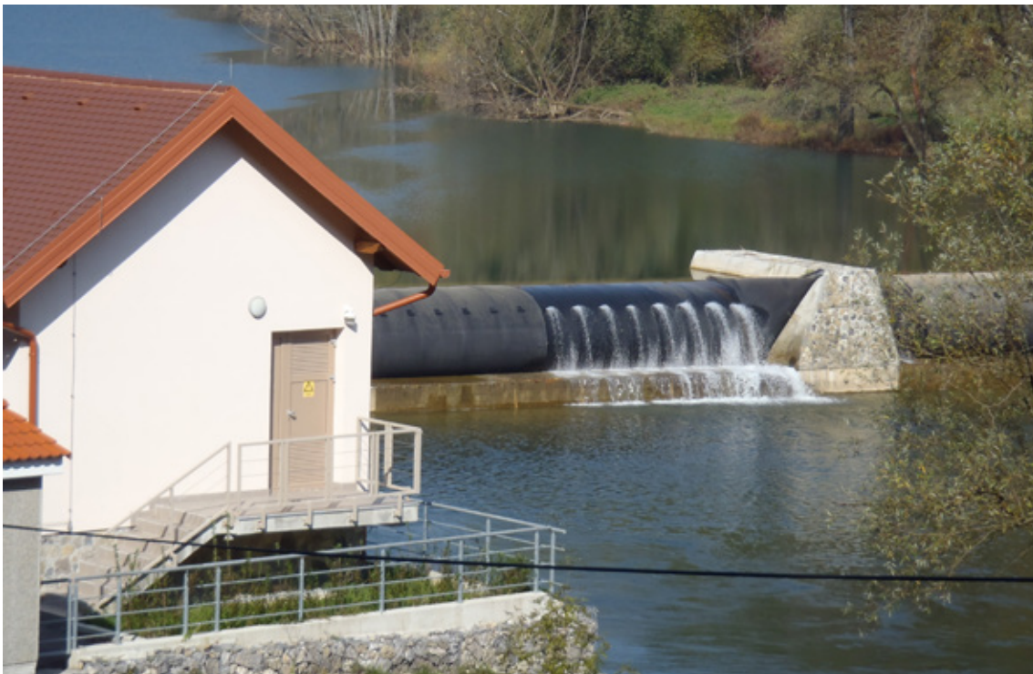
Figure 18: Ilovac dam, Croatia
