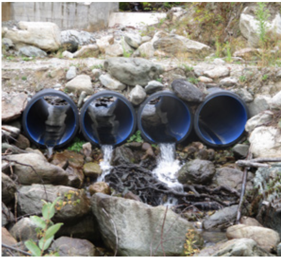
Figure 35: Culvert
