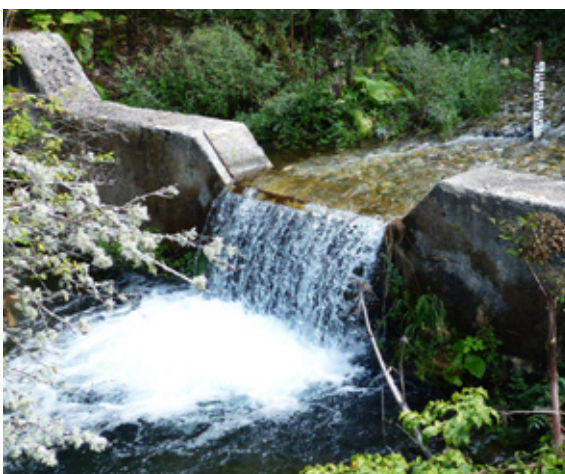
Figure 26: The weir above the powerhouse September 2017
